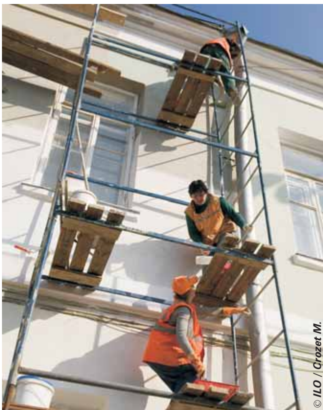
Building repairs at one of the central streets in Moscow (without proper security measures).
